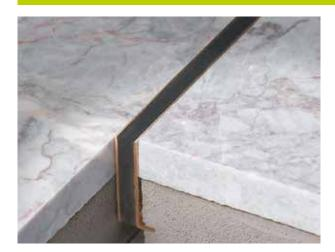
COFLEX CTM expansion joints are composed of a metal structure and a flexible yet durable central infill that can be ground and polished on-site. Due to their resistance to corrosion and wear, the profiles are ideal for resin-based terrazzo and natural stone tile installations. Ideally used in retail shops, hotels, sports facilities and schools.
